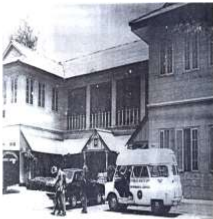
Public Health Offices, 43 Broad Street, Lagos, where the Late Dr. Isaac Ladipo Oluwole worked.
