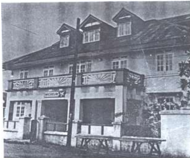
Late Dr. Isaac Ladipo Oluwole's house, 111, Griffith Street, Ebute-Metta, Lagos (Source: Society of Health Journal)
