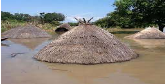
2012 Flood, Houses Submerged
